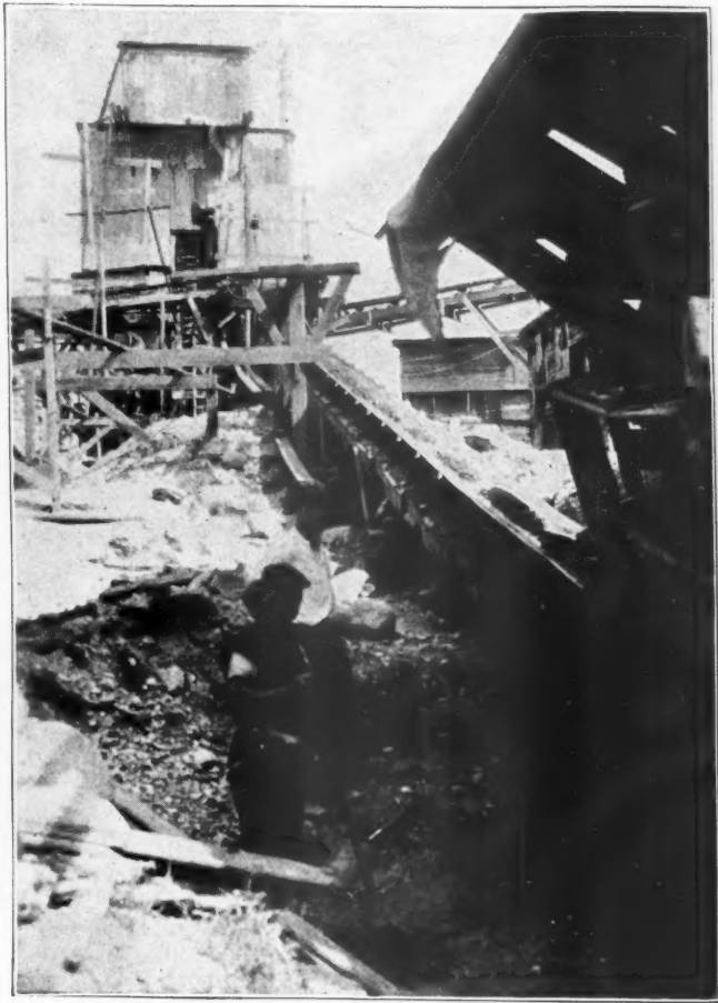
Conveyor From Hopper to Scalping Screen
